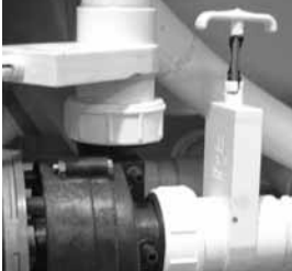
Slice Valve and Pump Union
